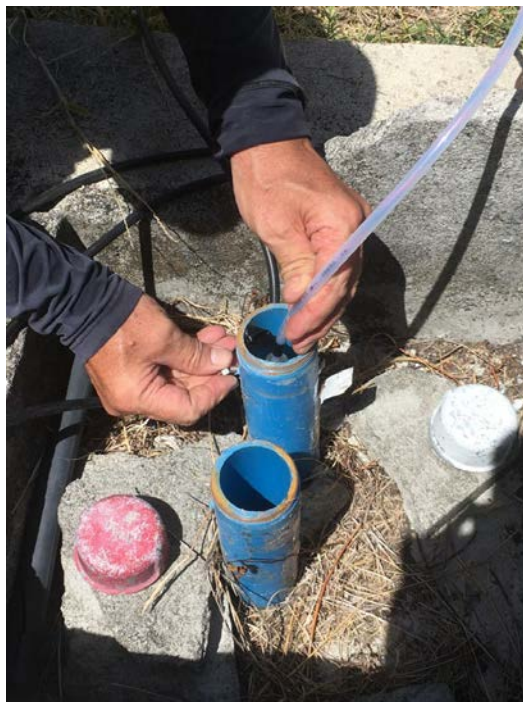
Figure 9. Installation of the water level sensor inside the injection well (P03)
