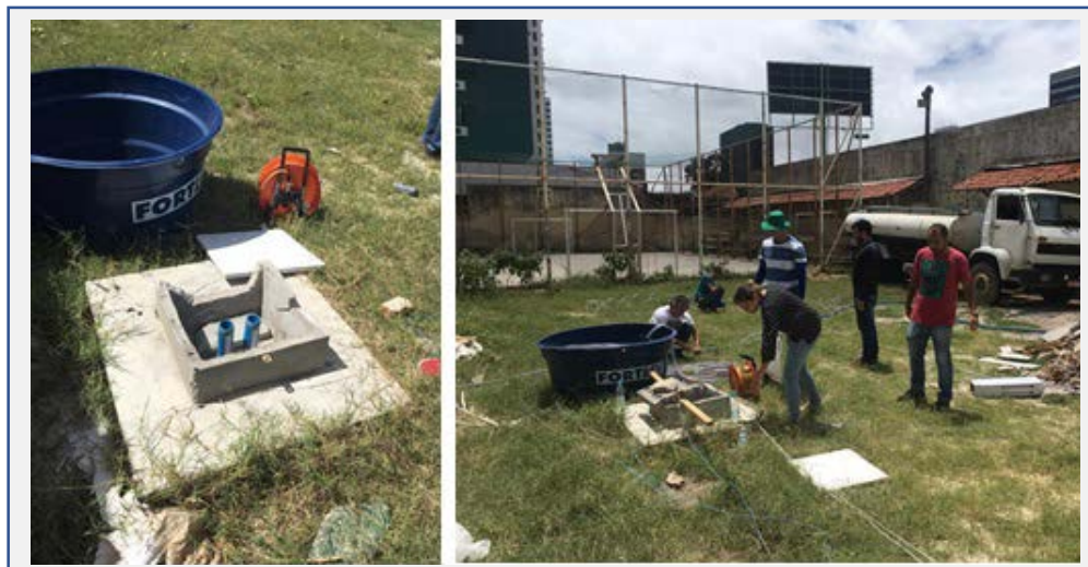
Figure 2. The area where the managed aquifer recharge pilot scheme is being installed - Pina, Recife, Brazil.
