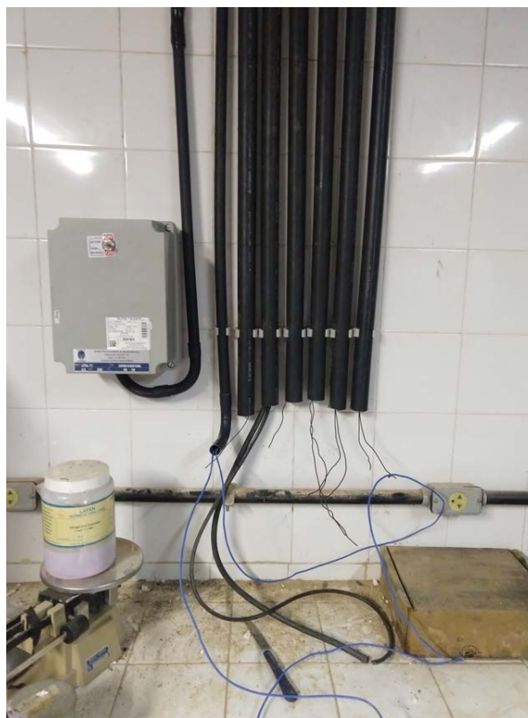
Figure 26. Drilling process – installation of pumping automation control & Ampeq monitoring system (source: SMART-Control project).
