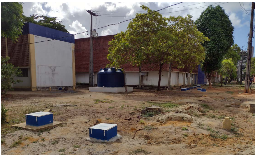
Figure 30. Drilling process – João Pessoa pilot scale overview after conclusion (source: SMART-Control project).
