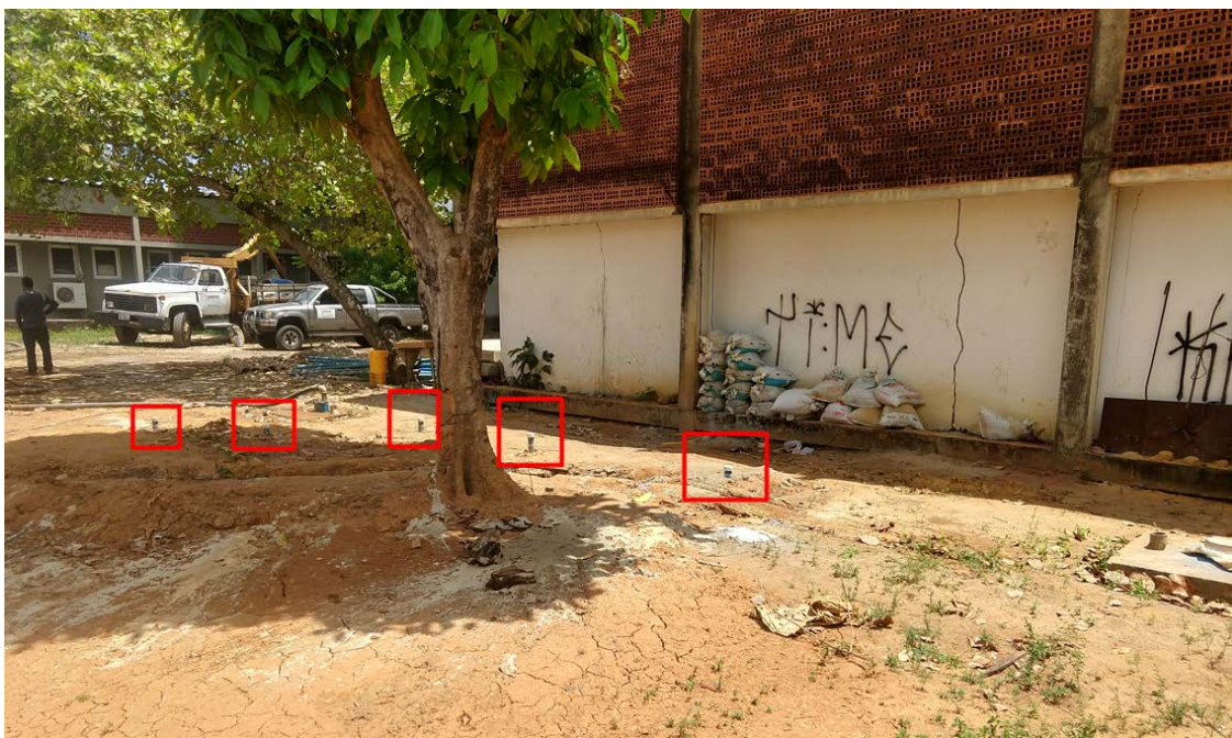
Figure 22. Drilling process – five new piezometers (source: SMART-Control project).
