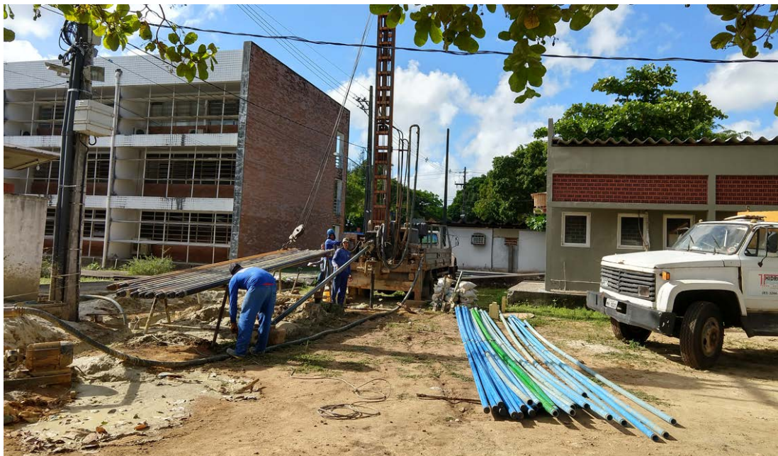
Figure 24. Drilling process – last two piezometers PZ-07 and PZ-08 (source: SMART-Control project).
