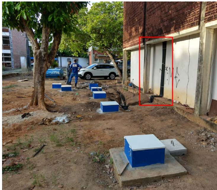
Figure 27. Drilling process – installation of tubes for Ampeq monitoring system (in red) and piezometers and well protection (source: SMART-Control project).
