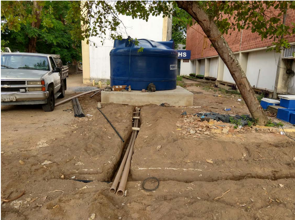
Figure 25. Drilling process – Installation of hydraulic facilities including storage tank (source: SMART-Control project).
