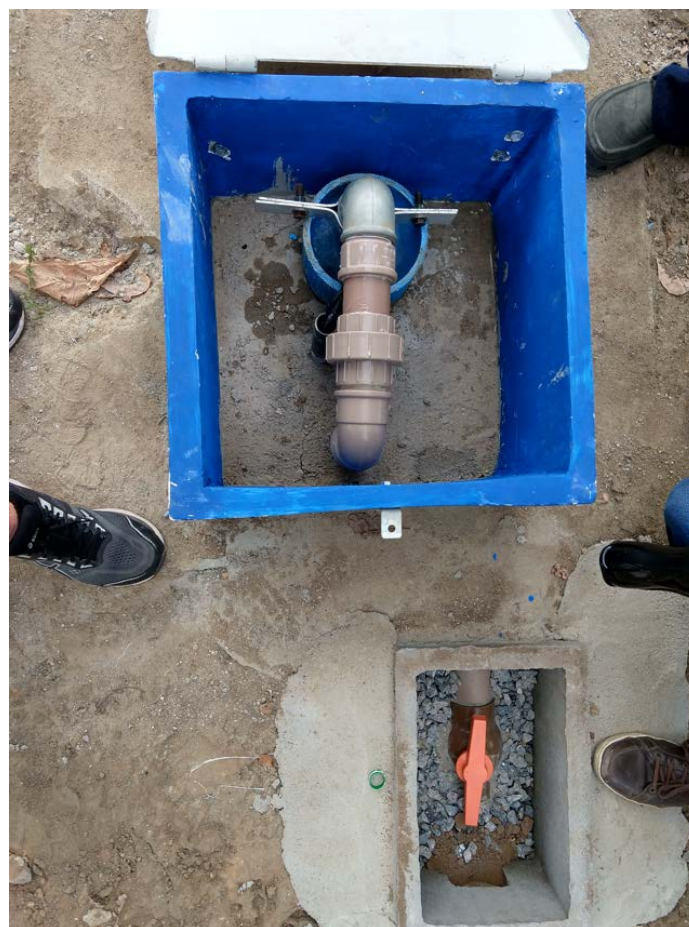
Figure 28. Drilling process – Pumping well and flow control valve (source: SMART-Control project).
