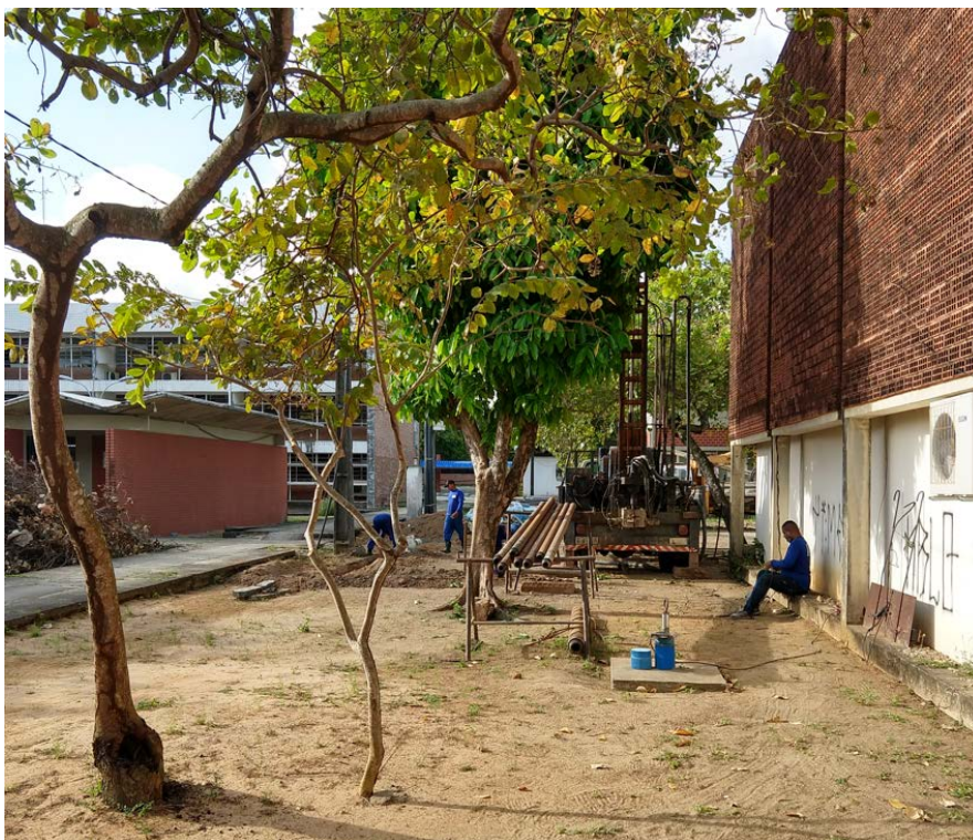
Figure 20. Beginning of the drilling process in the SMART-Control project and pre-existent injection well – PT-01 (source: BRAMAR project).
