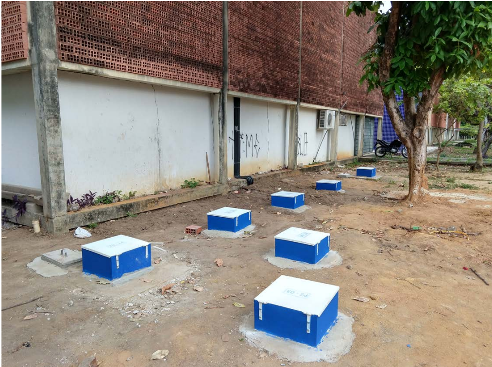
Figure 29. Drilling process – Conclusion of pumping and injection wells and piezometers (source: SMART-Control project).
