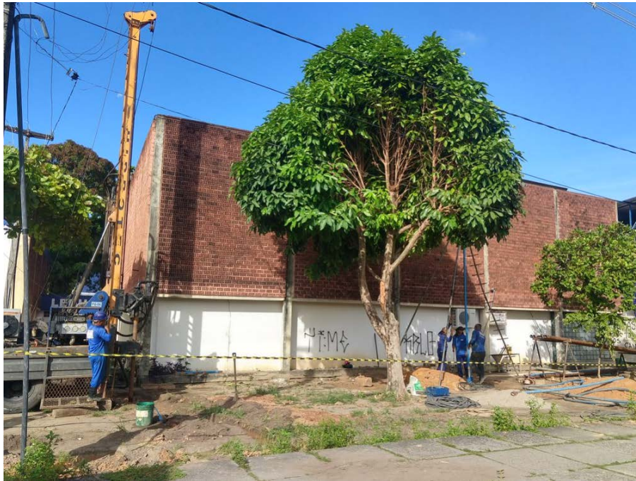
Figure 19. Beginning of the drilling process PT-01 (source: BRAMAR project).
