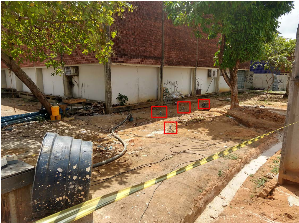
Figure 21. Drilling process – four new piezometers (source: SMART-Control project).
